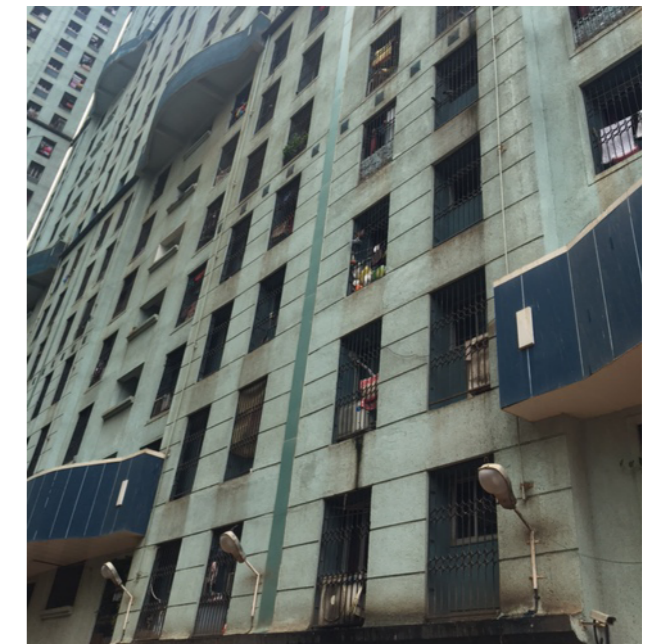
A photo of public housing in Mumbai. Photo Credit: Tanu Kumar.
